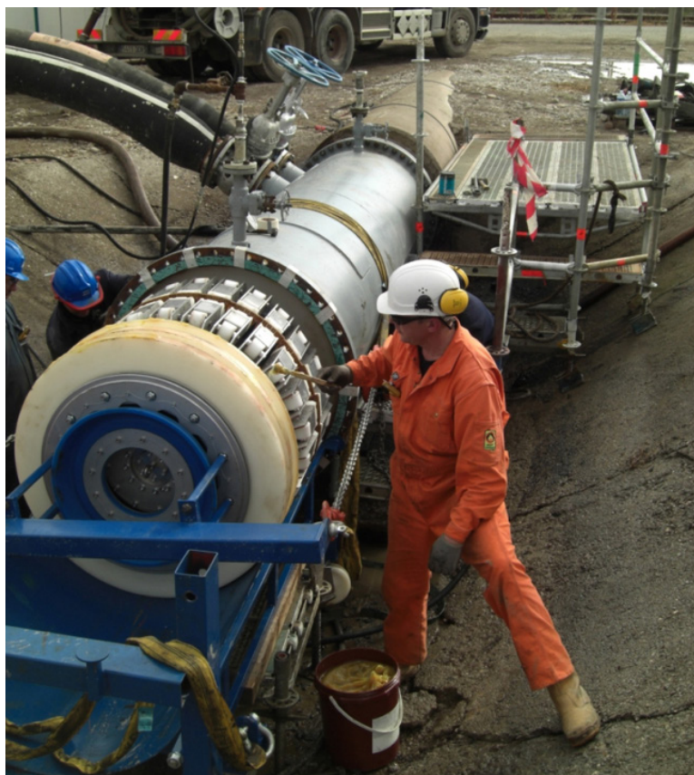
Figure 1. Launching a 42 in. bi-directional MFL tool into a marine terminal sea line.
